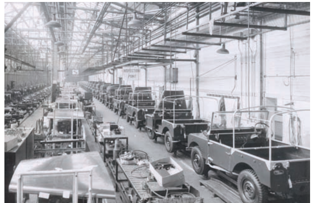
Above centre, left and right: A complete rolling chassis, correctly painted green, ready to leave Dunsfold for the recreated Series 1 production line at Solihull
